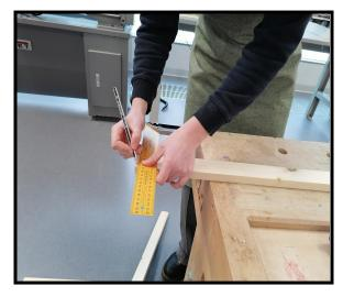
centimetre away. This is important because in the next step I sanded down the wood so that the edges were straight, the length was even for all planks used, and for safety to prevent potential splinters. After sanding I measured all the planks to guarantee they were uniform before I began to nail them together. I did this for four planks in total, two
